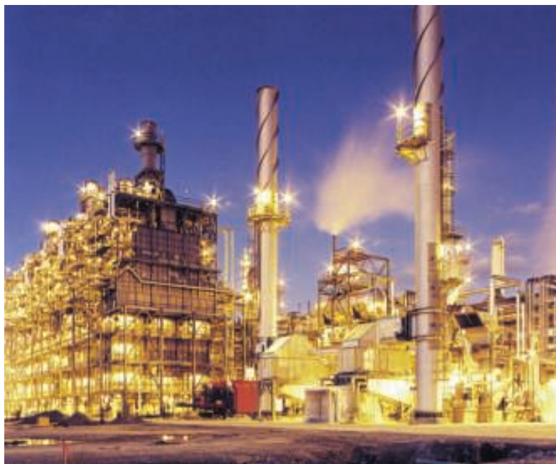
FIGURE 1. Safety should always be a priority at a process plant
