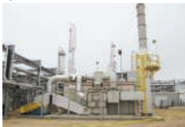
FIGURE 4. Regenerative thermal oxidizers provide a cost-effective-emission control solution as they achieve 99% destruction efficiency
